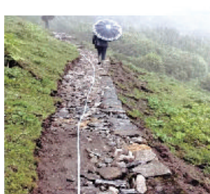
Shivadhara Infrastructure Development and Beautification Project in Makalu Rural Municipality, Ward No. 5
