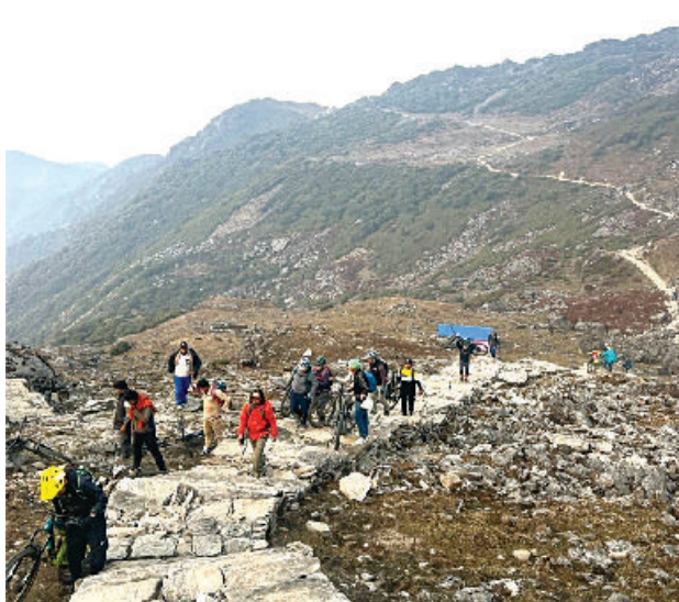
Bhairav Kunda Treking Trail Construction Project in Bhotekoshi Municipality, Ward No. 1 (Chhagam Bagam Site), Sindhupalchok
