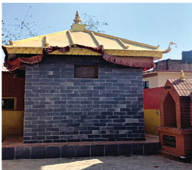
Jalpa Devi Temple Renovation Project in Kirtipur Municipality- 6, Kathmandu
